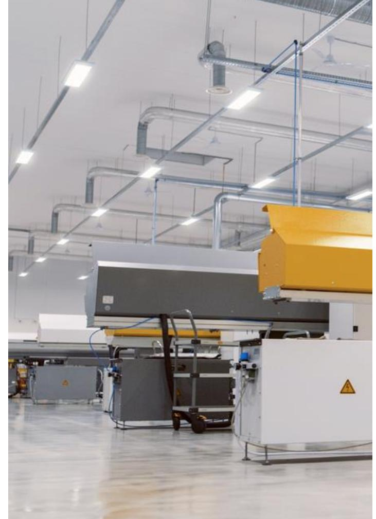
Luminary dedicated for big space industry areas. ceiling mounting. Light distribution made by using high performance lenses. Luminary body made from steel sheet, powder coated in white. The product is recommended for production halls, warehouses and heavy industry.
