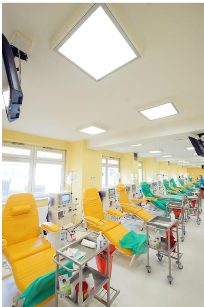
Dialysis station, hospital in Łomża
